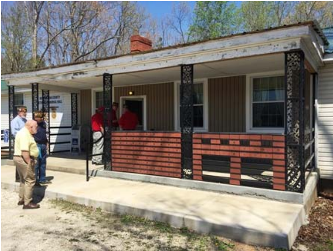
A unique wall at Buckingham Post 8446
