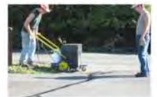
CRACK FILLING
